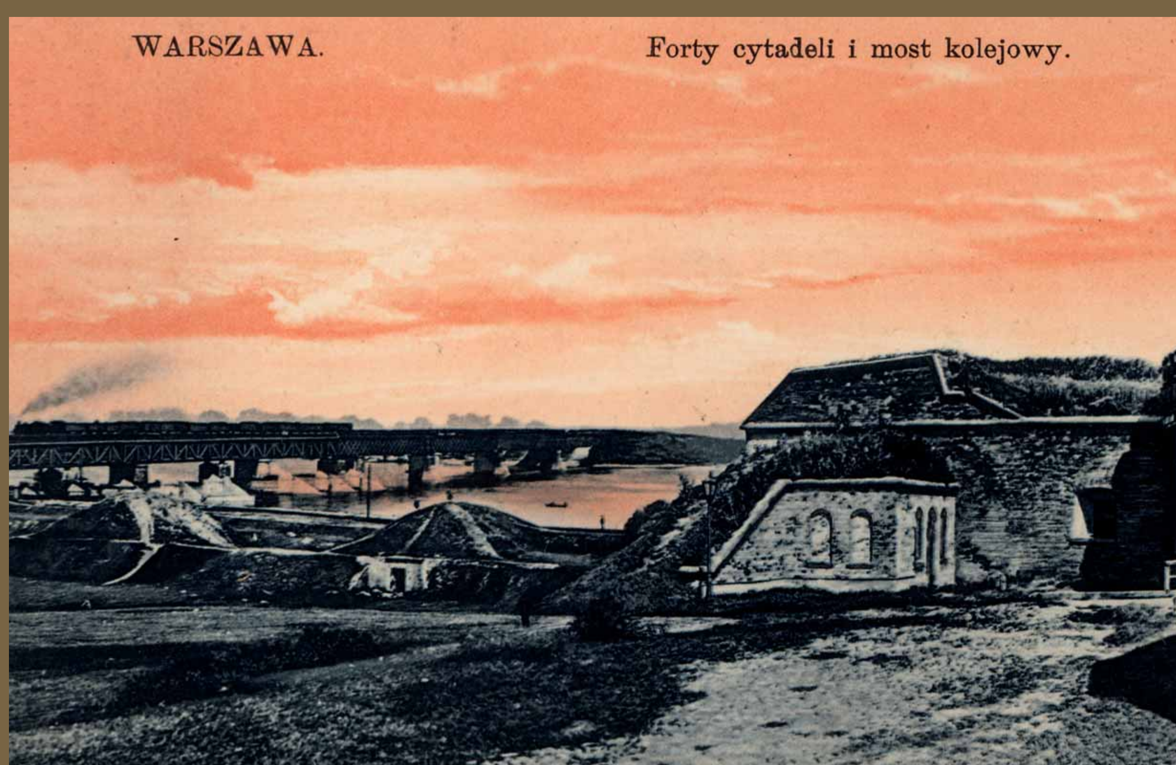
Most przy Cytadeli, b.d., 201/I-201 | Bridge at the Citadel, no date, 201/I-201
