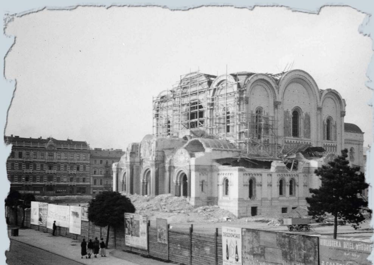
Rozbiórka cerkwi Aleksandra Newskiego w Warszawie ( Demolition of the Alexander Nevsky Cathedral in Warsaw, belonging to the Eastern Orthodox Church ), 1924–1926, 72/1630/2017
