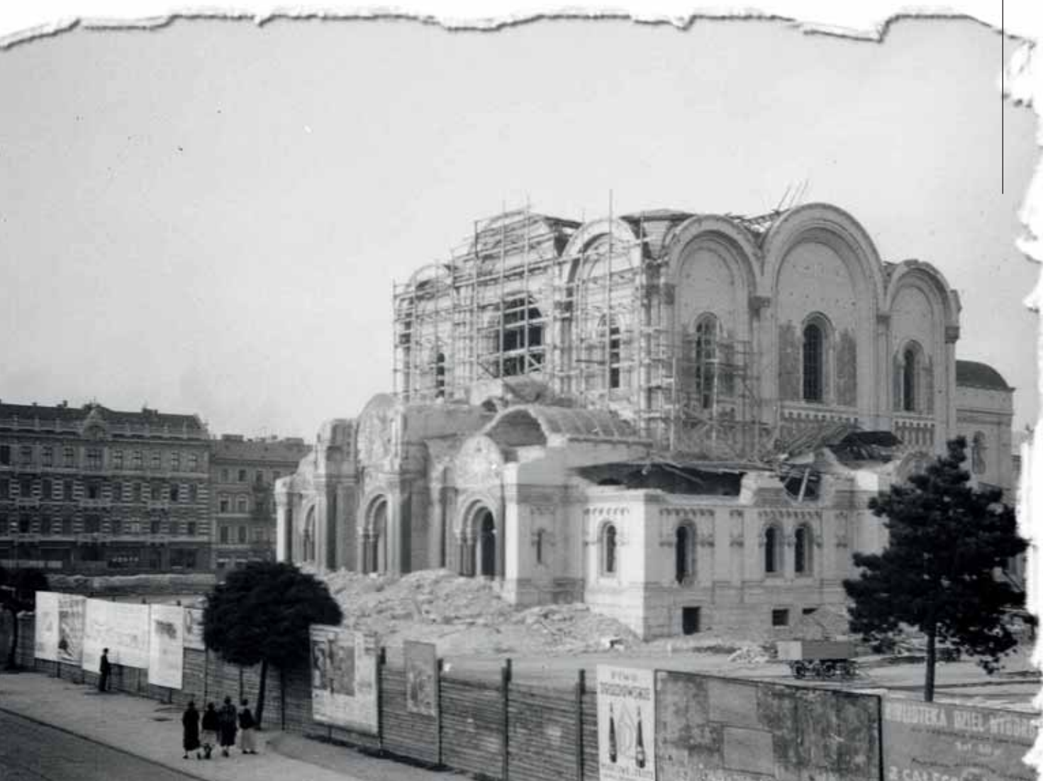
Rozbiórka cerkwi Aleksandra Newskiego w Warszawie ( Demolition of the Alexander Nevsky Cathedral in Warsaw, belonging to the Eastern Orthodox Church ), 1924–1926, 72/1630/2017
